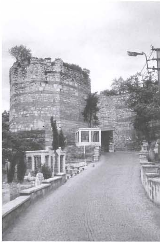
Plate 41 Kaligaria Gate, outer (western) view
